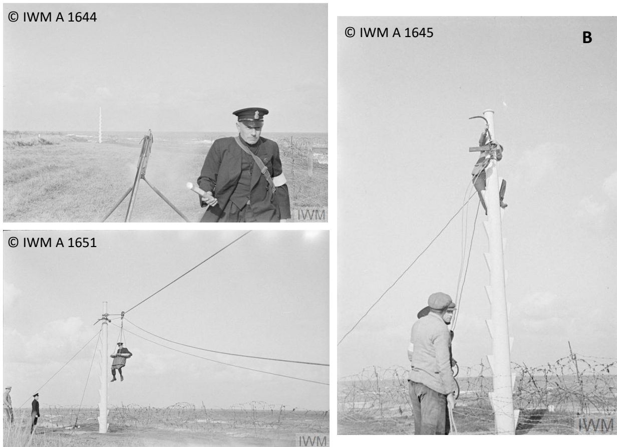
Figure 22. A. Rocket pole on concrete mount at The Station, Lower Whitehall ( https://scapetrust.org/sites-at-risk/site/16201 ); B. Rocket apparatus in use in practise in Happisburgh, Norfolk in 1940. The rocket fires a line to the ship's mast (the pole) and a breeches buoy is set up to rescue the crew. © Imperial War Museum.
