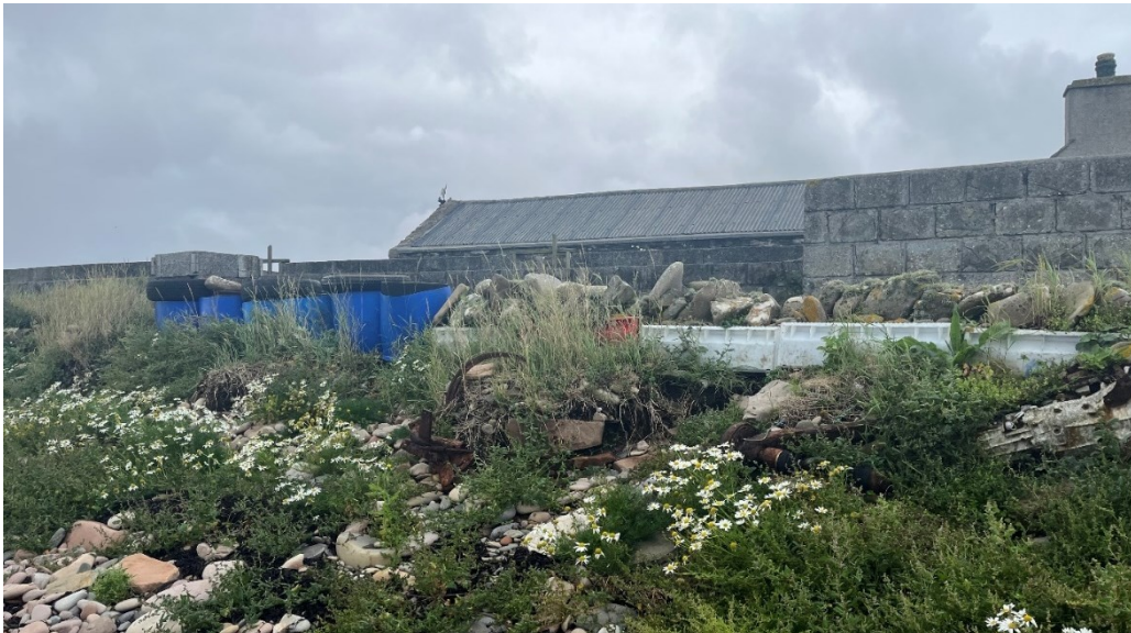
Figure 11. Ad-hoc coastal defences protecting farm buildings at Furrewend
