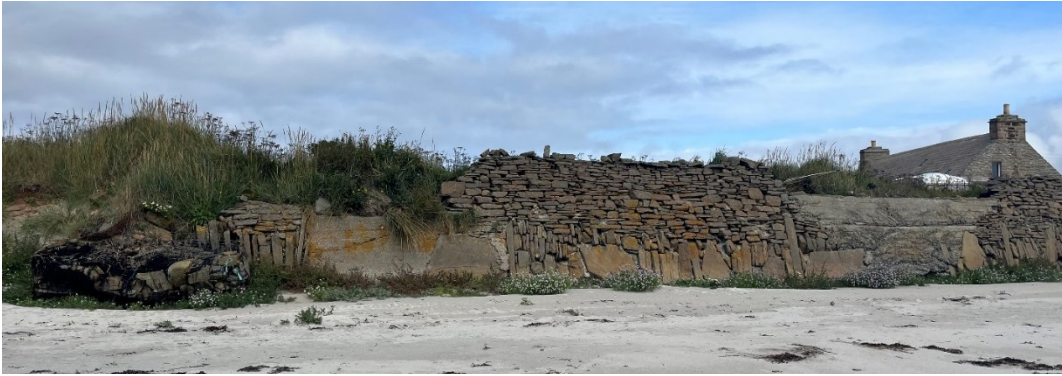
Figure 12. Multi-phase coastal defence at Banks.
