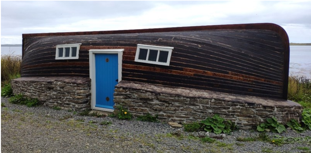
Figure 31. Wash house with roof made from lifeboat ( https://scapetrust.org/sites-at-risk/site/16192 ).
