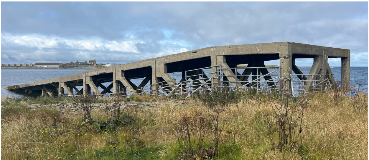
Figure 19. The Station concrete lifeboat slipway, built in 1911 ( https://scapetrust.org/sites-at-risk/site/16203 ).
