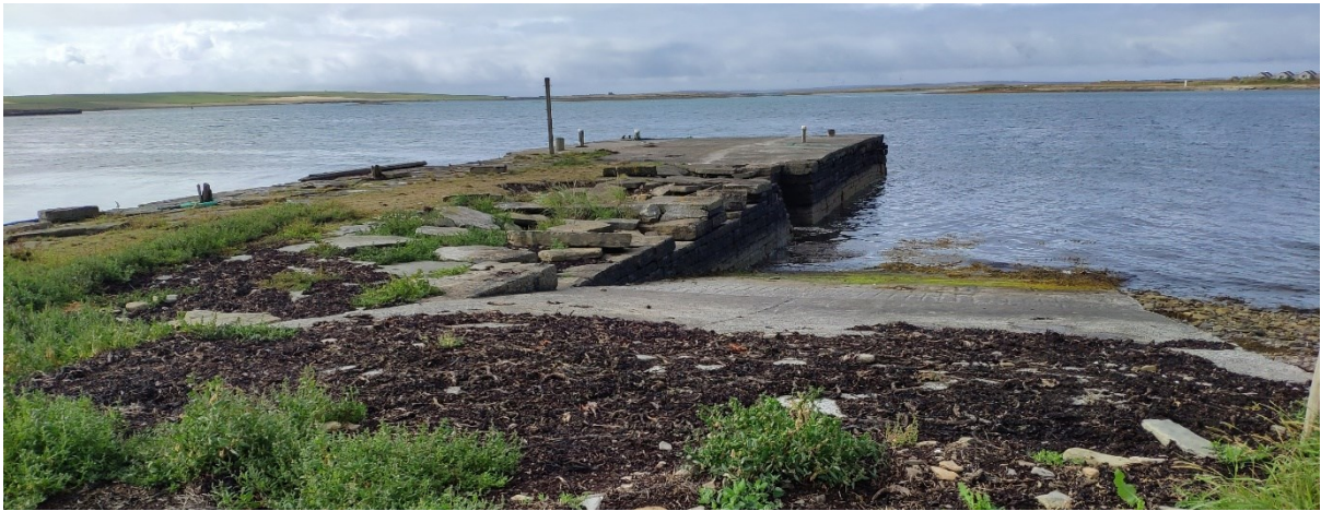
Figure 18. The Station Pier, and an adjacent concrete slipway. The Station Pier was built in the late 1800s for the herring fishing industry and the concrete slipway was built by the Monks living on Papa Stronsay as a landing place for their small craft ( https://scapetrust.org/sites-at-risk/site/16084 ).
