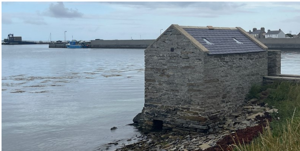
Figure 36. Small stone built tidal toilet located on the coast edge. Built for, and used by, workers in the herring industry ( https://scapetrust.org/sites-at-risk/site/16193 ).
