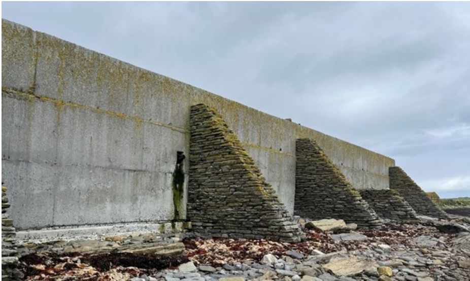
Figure 13. large concrete and stone built coastal defence for Houseby Farm.
