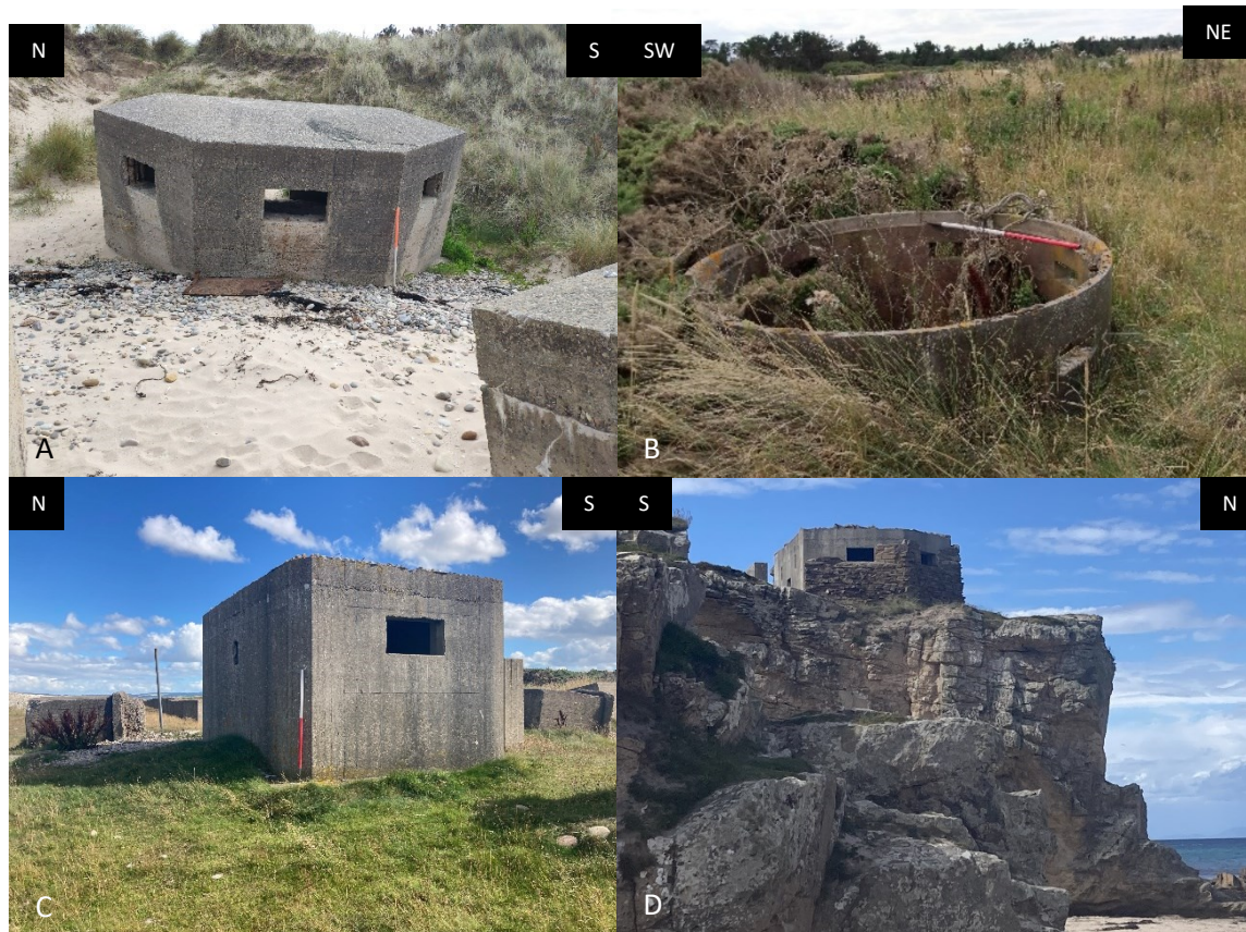
Figure 19. Examples of pillbox styles along the Moray coastline. (A) Type 24 six-sided pillbox, Burghead Bay ( https://scapetrust.org/sites-at-risk/site/14342 ); (B) Round Norcon style pillbox, Spey Bay ( https://scapetrust.org/sites-at-risk/site/15650 ); (C) Medium machine gun rectangular pillbox, Innes Links ( https://scapetrust.org/sites-at-risk/site/14259 ); (D) Type 24 pillbox camouflaged with added stone cladding, Covesea Links ( https://scapetrust.org/sites-at-risk/site/14294 ).
