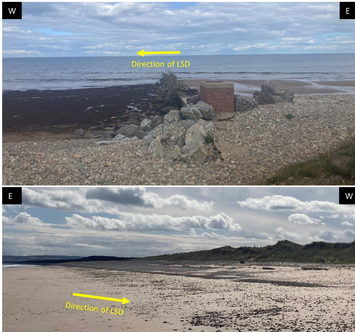
Figure 5. (A) Sewage pipe demonstrating westerly direction of longshore drift (LSD) of sand and shingle towards Spey Bay with a larger quantity and higher level of gravel on the eastern side of the pipe than on the western side. The pipe is defended using rock armour and gabions; (B) Transition between shingle and sand just east of Lossiemouth. Direction of LSD from east to west. At the time of the CCZAS in August 2022, the transition from the shingle dominated sediment originating from the Spey to the predominantly sandy beaches to the west, occurs at BNG 325270 869580.
