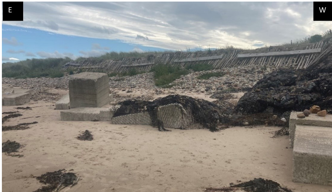
Figure 13. The edge of the golf course was re-profiled in November 2021 and wooden fencing anchored to the base of the section. There are also the remains of failed gabions and tumbled anti-tank cubes.
