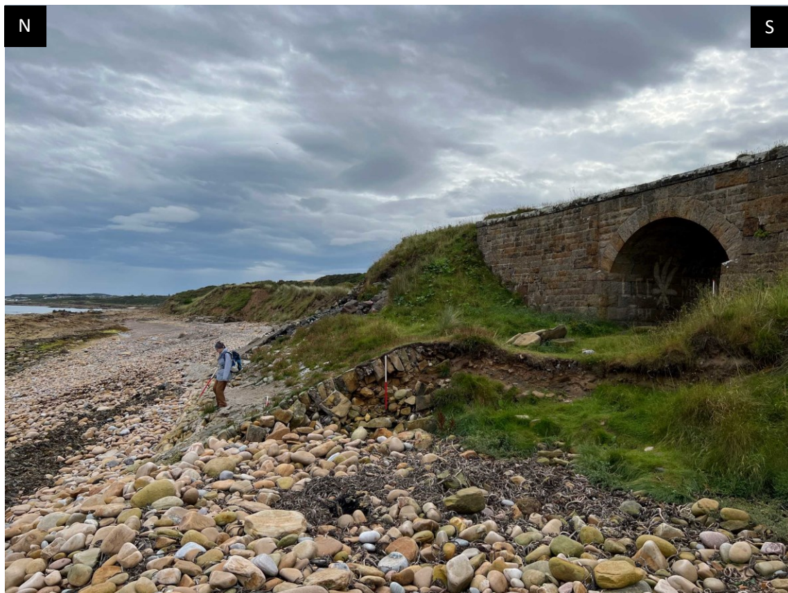
Figure 11. Eroded embankment of Burghead Railway in foreground and background
