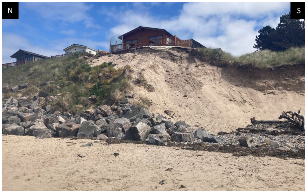
Figure 10. Erosion of sand dune coast edge at chalet part to the east of Burghead Bay. Eroding 'bite' at the end of the rock armour.
