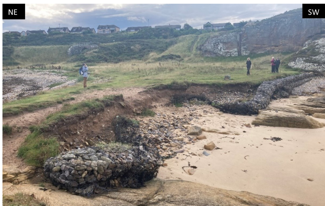
Figure 12. Example of coastal defence which has failed, Cummingstown.
