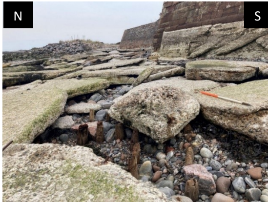
Figure 10A. Concrete landing platforms on northern side of Fort George showing heavy deterioration due to coastal erosion, revealing wooden supporting posts underneath.
