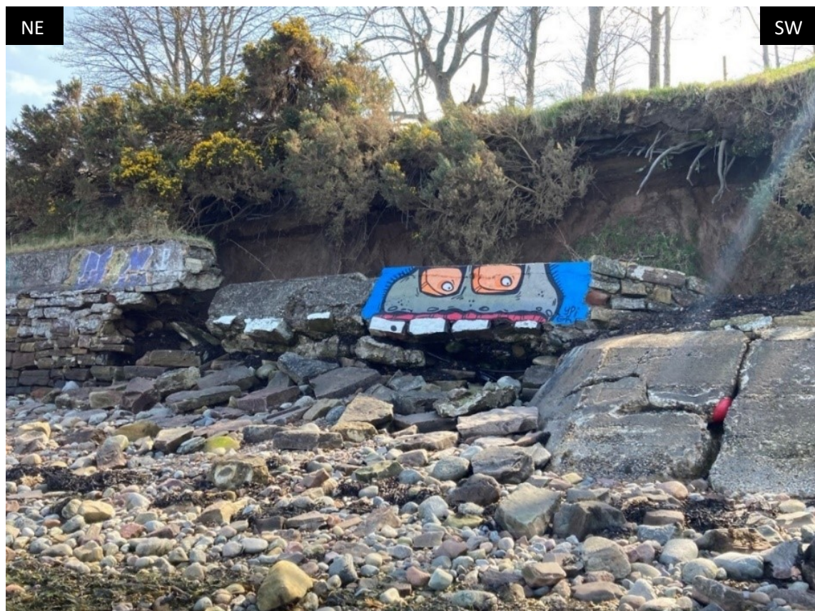
Figure 5. Damaged stone and concrete embankment at Milton of Culloden protecting soft sediment coastline behind
