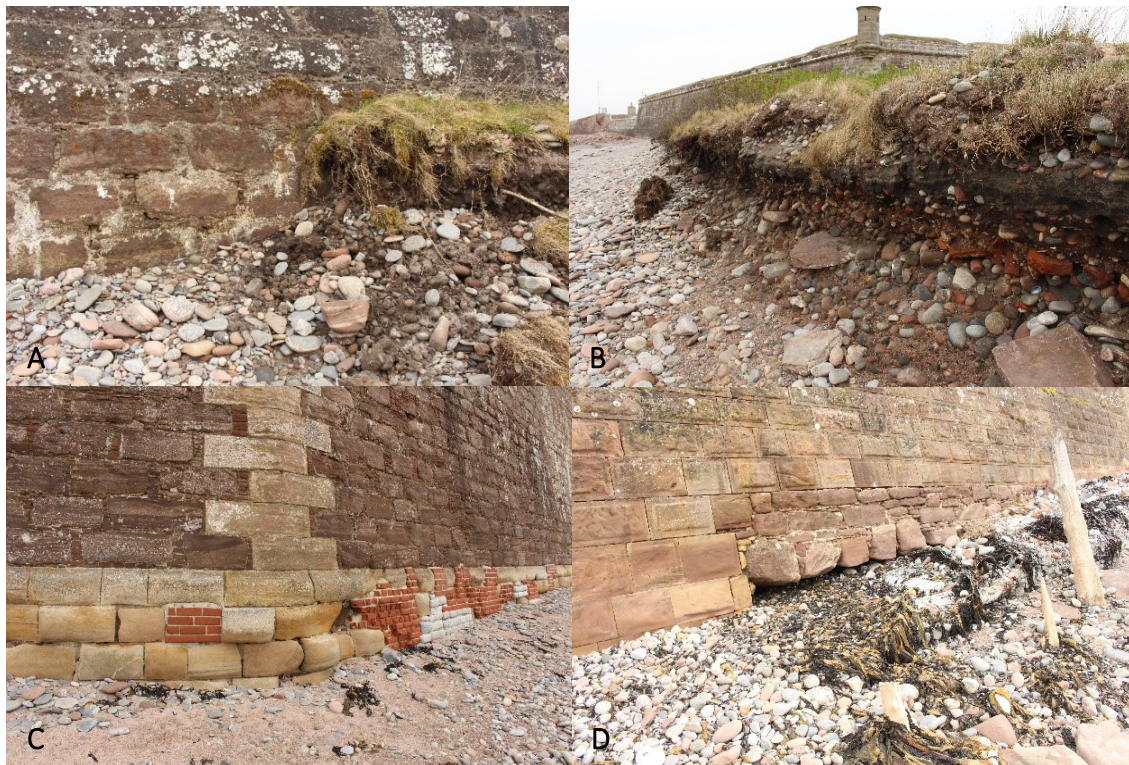
Figure 9. (A) Level of previous level of sediment is noted by colour variation in stonework, northern side of Fort George outer walls. Cherry-cocking dressed stone below sediment level suggests that wall has been exposed before. (B) Active erosion and undermining of sediment, on northern side of Fort George, to the west of the dog cemetery. (C) Repairs that have been made to base of outer wall. (D) Repairs to outer wall and damage at current gravel beach level. Wooden posts suggest past attempts of sediment stabilisation.
