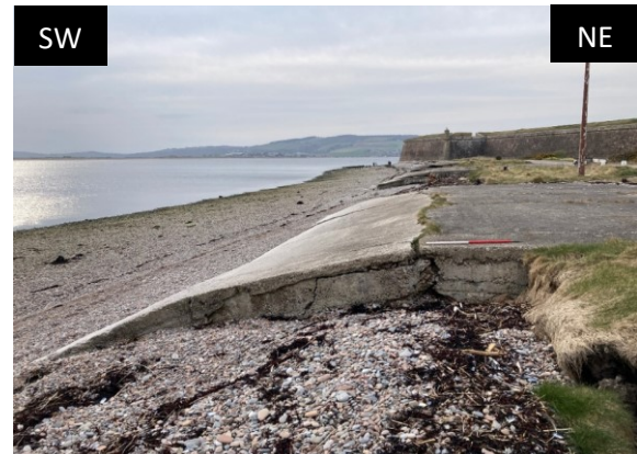
Figure 10B. Concrete landing platforms on the southwestern side of Fort George which are showing signs of deterioration.
