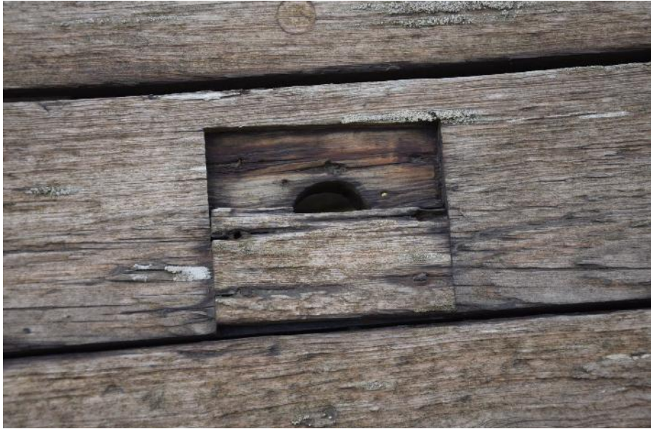
24. Patched setting in deck planking for structure / equipment
