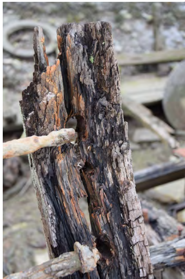
13. Bolt holes for chainplate in second port bow frame
