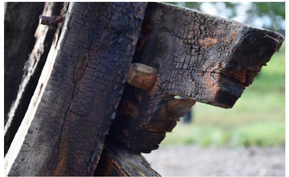
27. Interior side of patch showing wooden pin
