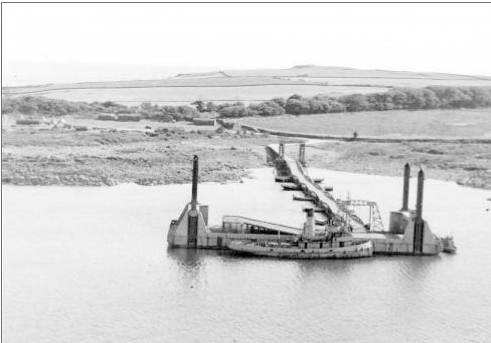
Figure 28. Contemporary photograph of the Mulberry Harbour floating roadway design during sea trials at Cairnhead, with the accommodation camp and service buildings in the background. The pontoons supporting the roadway are visible, one survives on site (13904). From http://www.mulberryharbour.info/ , picture credit IWM.
