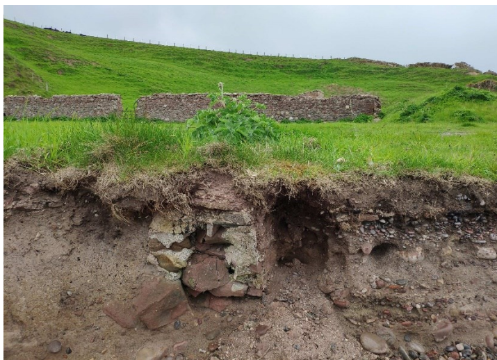
Figure 7A. Mortared stone wall eroding out of coast edge, Pennan Mill Bay ( https://scapetrust.org/sites-at-risk/site/15529/ ); B. Comparison of modern coast edge aerial photography from 2021 (@Getmapping Plc, 2023) and National Grid 1:2500 1 st Edition mapping from 1969-70 (Crown Copyright 2023, EDINA supplied service). There has been ~9m of coastal erosion in the last 50 years.
