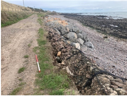
Figure 4A. Hard coastal defences in the form of rock armour and gabions. Evidence of failure of gabions, Seagreens, Aberdeenshire.
