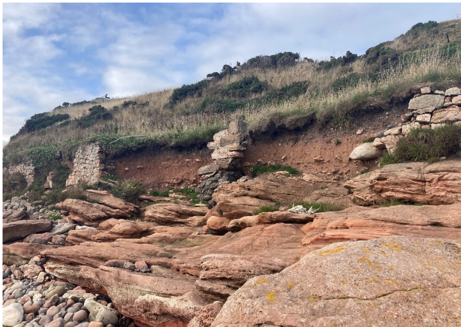
Figure 4C. Erosion of revetment wall, Seagreens, Aberdeenshire.
